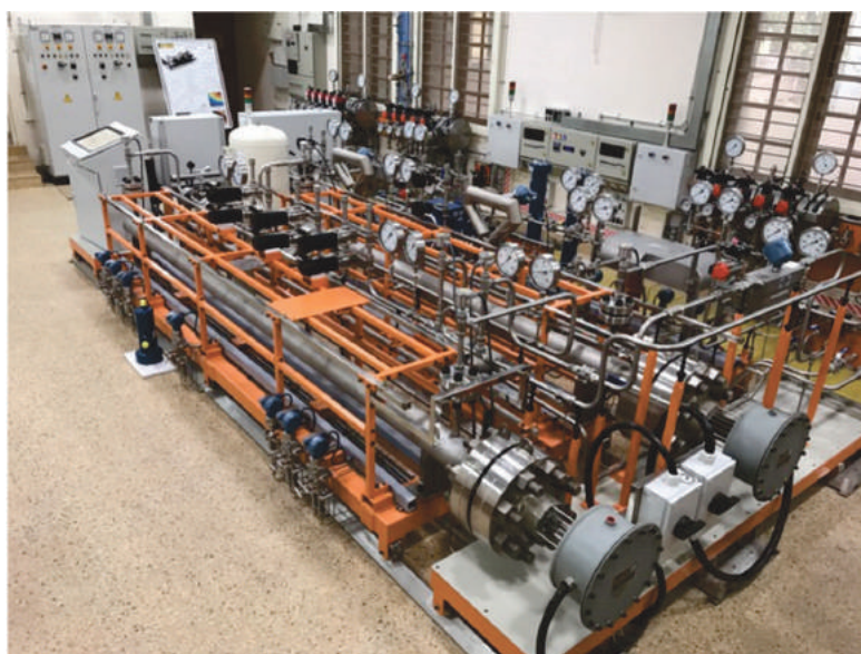
Supercritical CO 2 Brayton Cycle Test Facility at IISc Bengaluru
