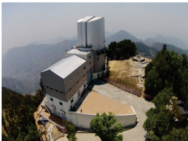
3.6m Devasthal Optical Telescope (DOT) Building.
