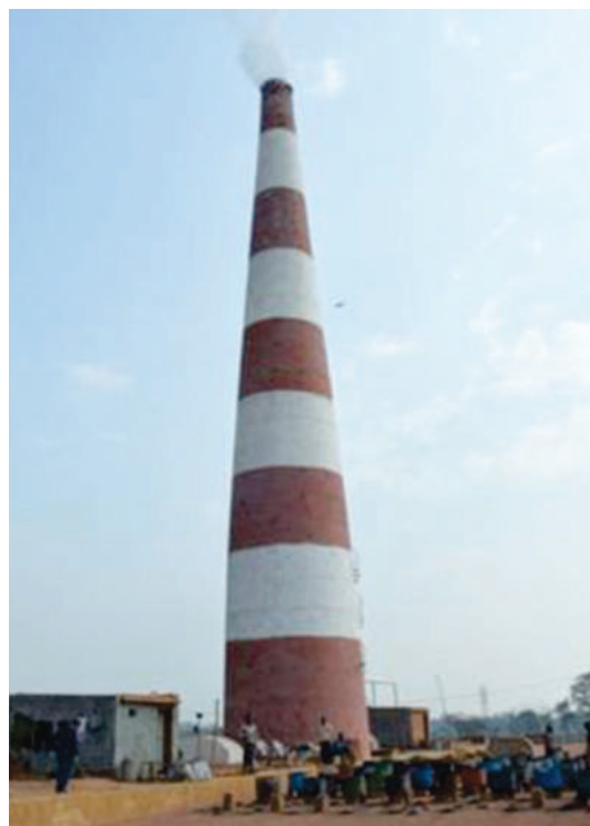
New Hybrid Kiln with zig- zag technology
