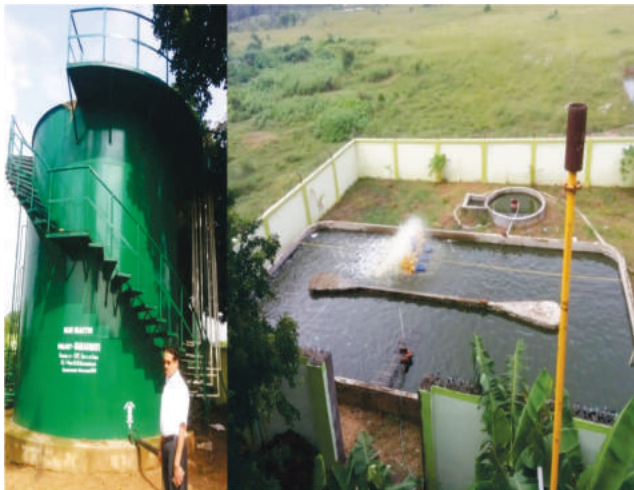
Anaerobic and natural treatment plant for black-water treatment, Kharagpur, West Bengal (IIT Kharagpur and CENTA, Spain)
