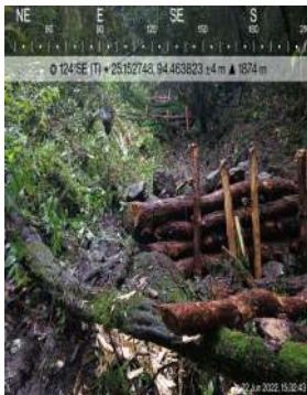
Fig. Crib Structures at the spring site
