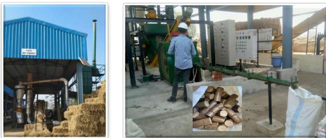
Fig. Paddy Straw briquetting plant at M/s PRESPL, Village Kulburchan, Distt. Patiala, Punjab, established in Public Private Partnership (PPP) mode.
