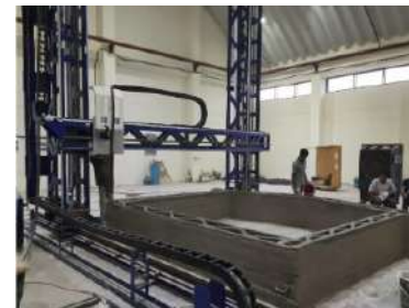
Fig. 3D Concrete printer
