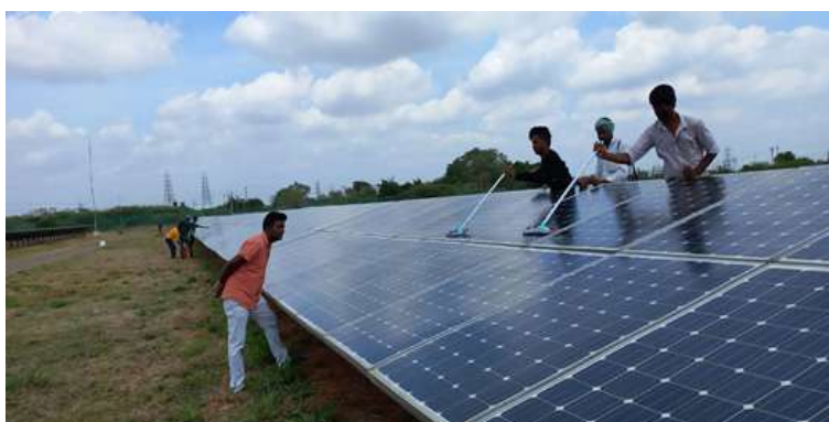
Fig. ARCI's Easy-to-clean coating technology deployed at a PV plant with 600 KW capacity at BHEL, Trichy.
