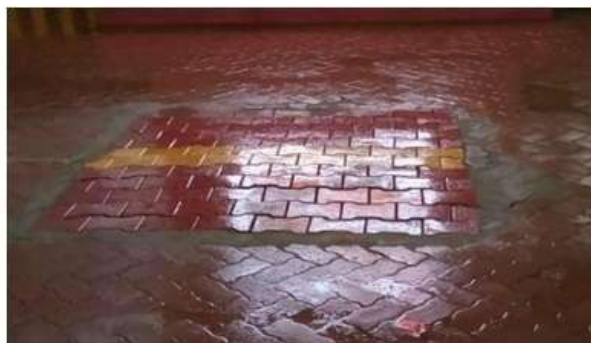
Fig. Red mud containing geopolymer pavers laid on a pathway
