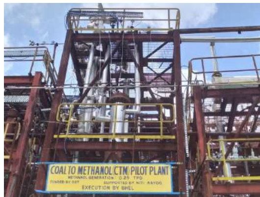
Fig. Indigenously developed 0.25 TPD Coal to Methanol (CTM) Pilot Plant by BHEL, Hyderabad
