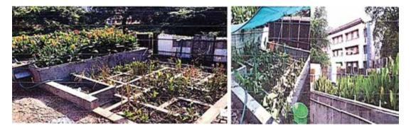
Figure. 10. Integrated domestic wastewater treatment system with multi-species and dual media constructed wetland
