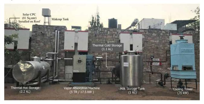
Schematic of the Solar Thermal Assisted Rapid Bulk Milk Cooler
